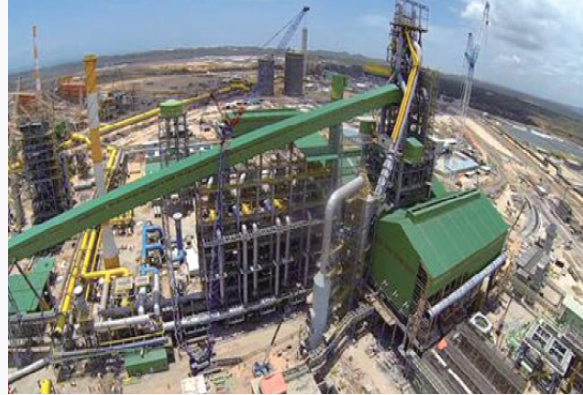
BRAZIL CSP STEEL PLANT PJT
